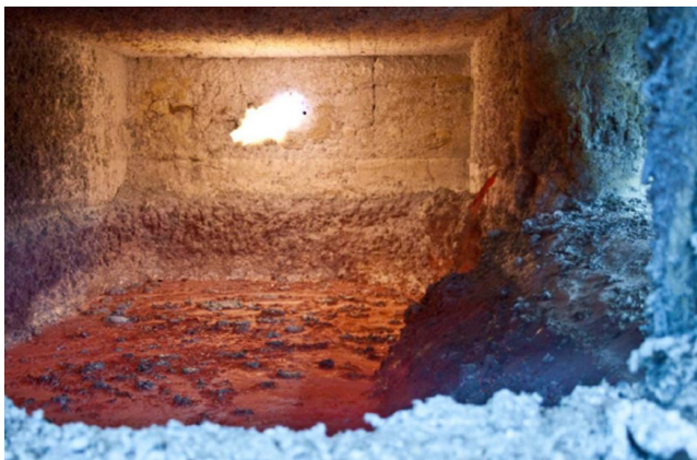
Furnace appearance before rebuild
