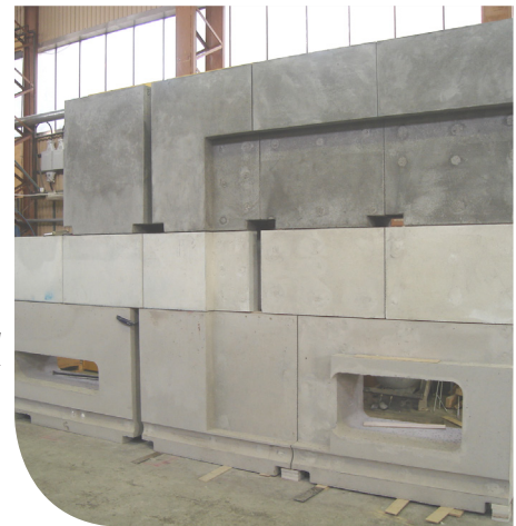
Rebuild was performed using Pyrotek precast furnace shapes
