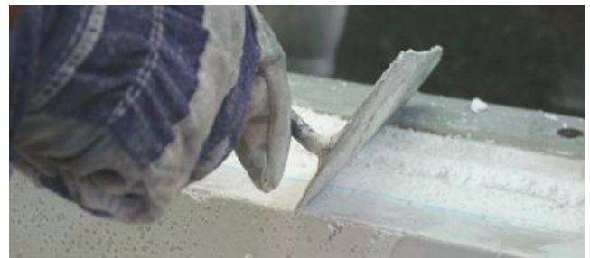
Trimming Excess Material
